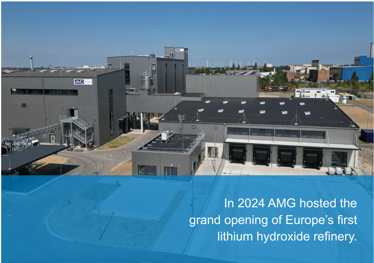
Lithium Hydroxide battery-grade refinery (Bitterfeld, Germany)
